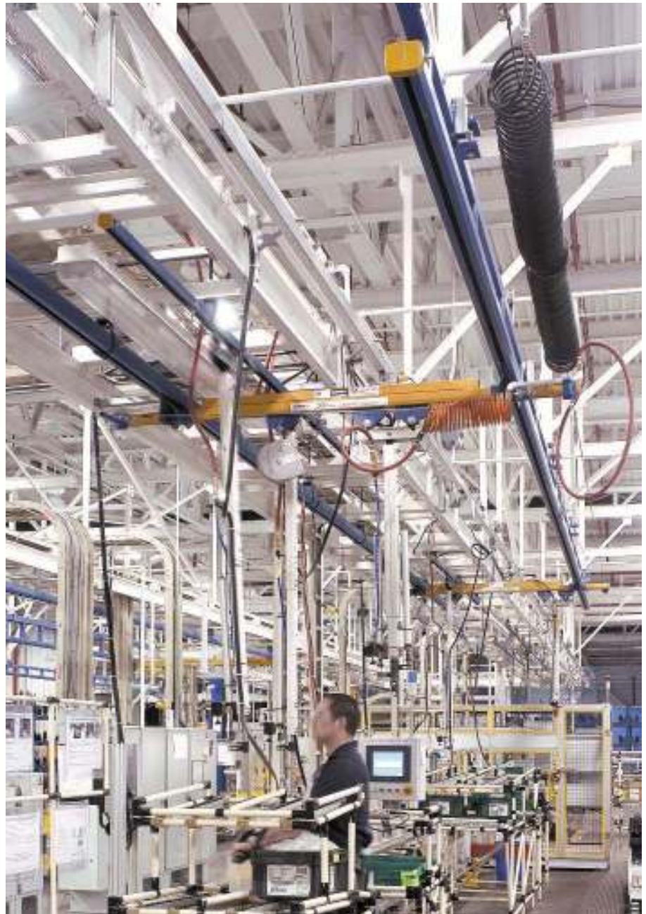
GM's St. Catharines, ON, V6-engine plant is using Gorbelt overhead cranes with impressive results.
