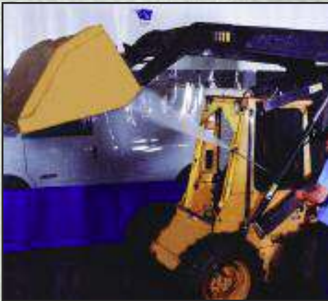
Curtains Provide Protection From High Pressure Overspray
